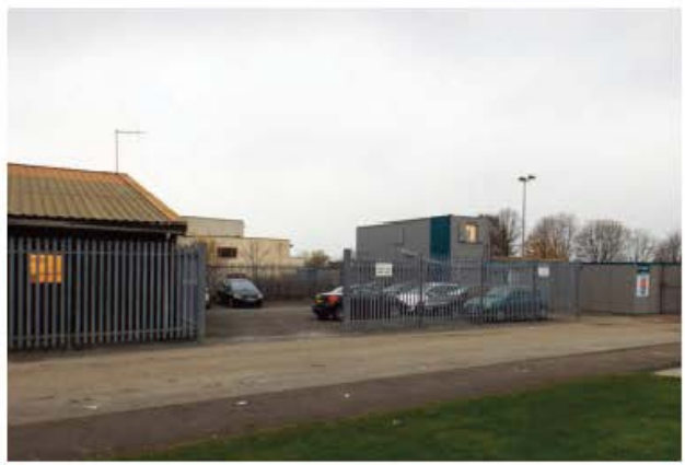
View of site office and Staff Car Park of advice centre
